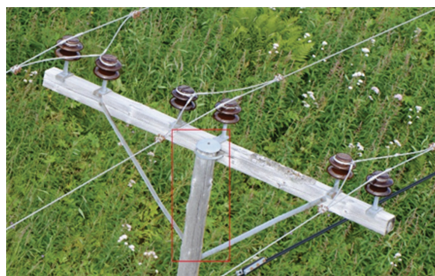
Figure 7. Wooden pole where a crack has been localized on the mast (see rectangle).
